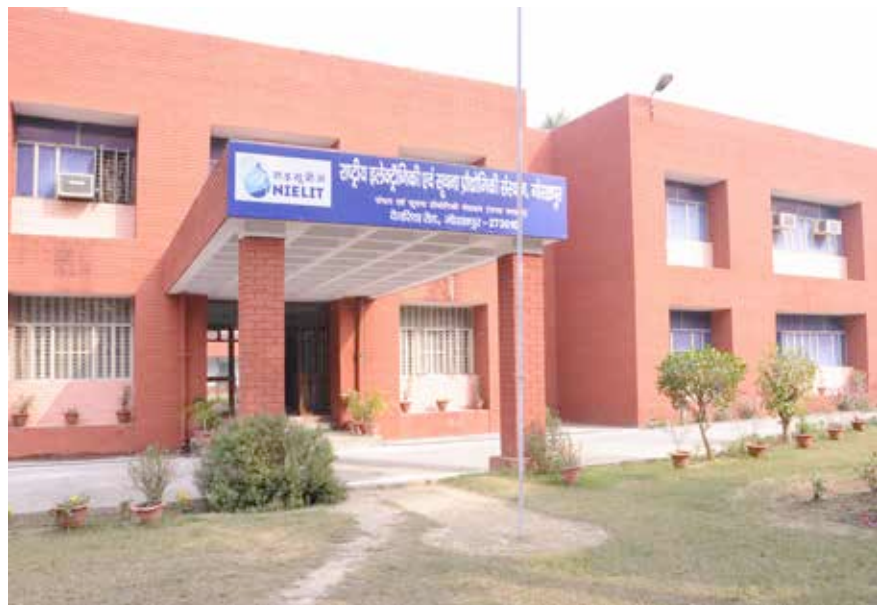
The building of National Institute of Electronics & Information Technology (NIELIT) Gorakhpur.
