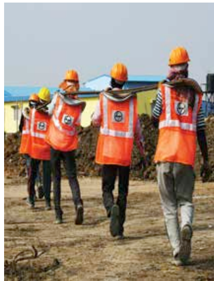
Work on a smart city project in progress
